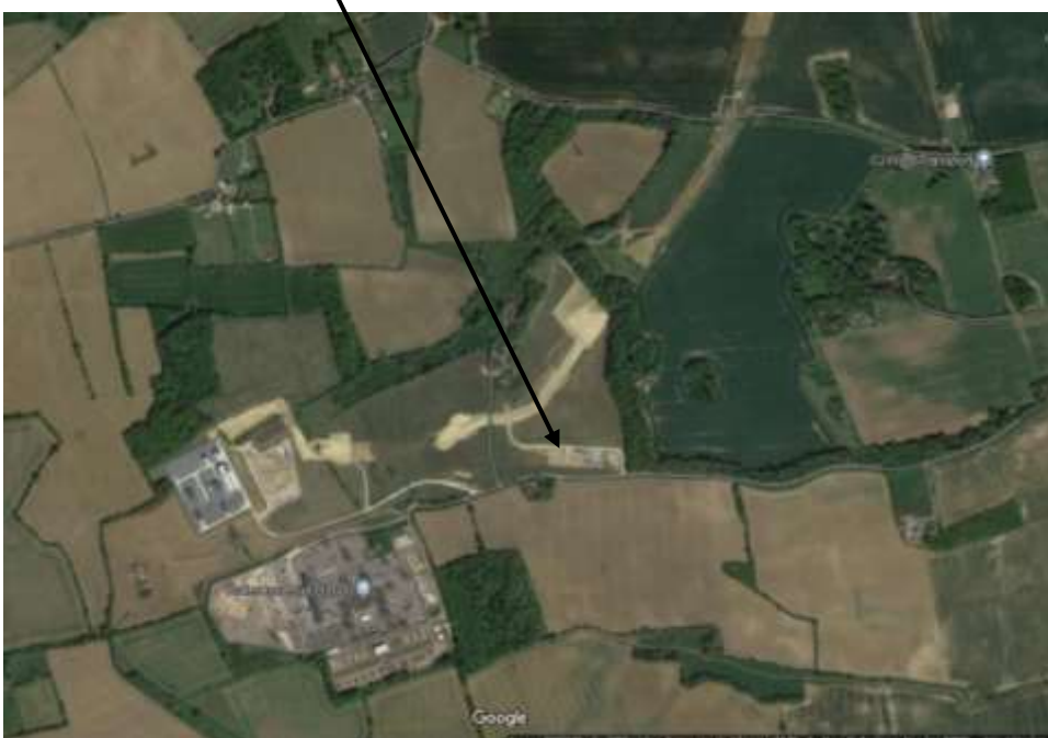
EA1 & EA3 cable site compound
